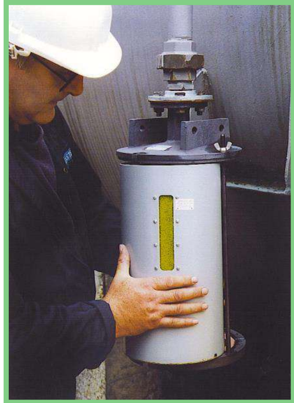
Transformer Breathers can be changed in a matter of minutes with Brownell's replacement cartridges. (Size W illustrated)
